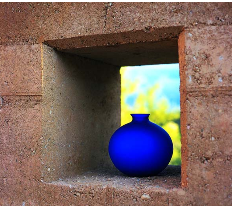
Rammed-earth wall (Woodin Construction).
